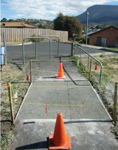
Figure 4 - The World's First Eco-Cement Porous Pavement, Windsor Park, Glenorchy, Tasmania
